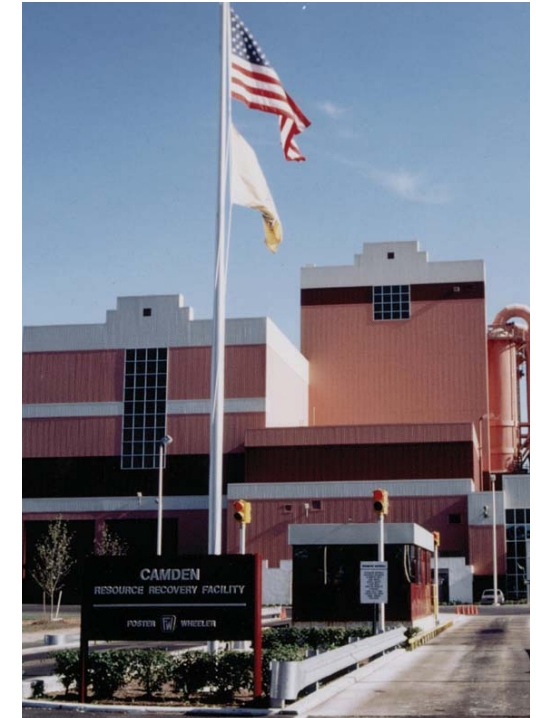
Camden County Energy Recovery Plant, 22 MWe
