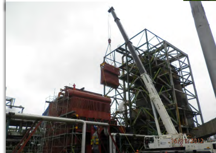
Boiler Substitution CB2 Madero Refinery
